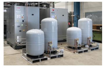
A contained ethane/propane cascade cooling system
